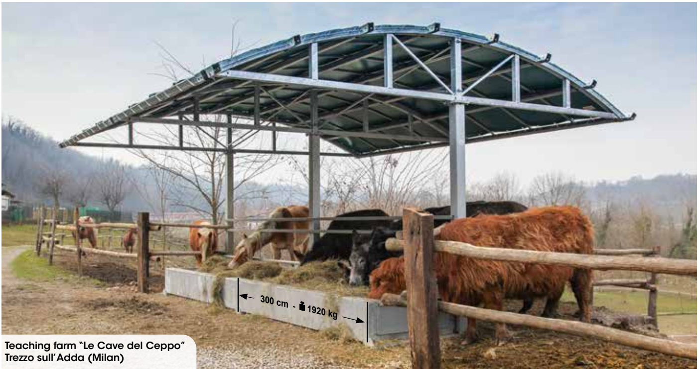
2-module shed - length: 600 cm. Roofing: class 2 flameproof PVC tarpaulin (colour: green)
